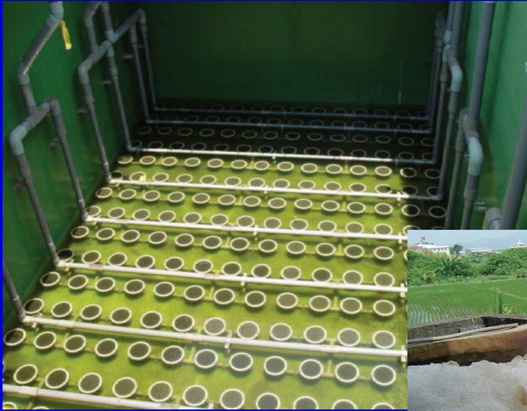
曝氣槽散氣盤安裝
